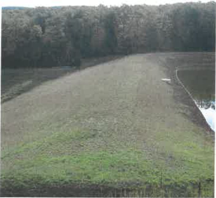
WILSON DAM MODIFICATION, HAMPSHIRE CO., WV
