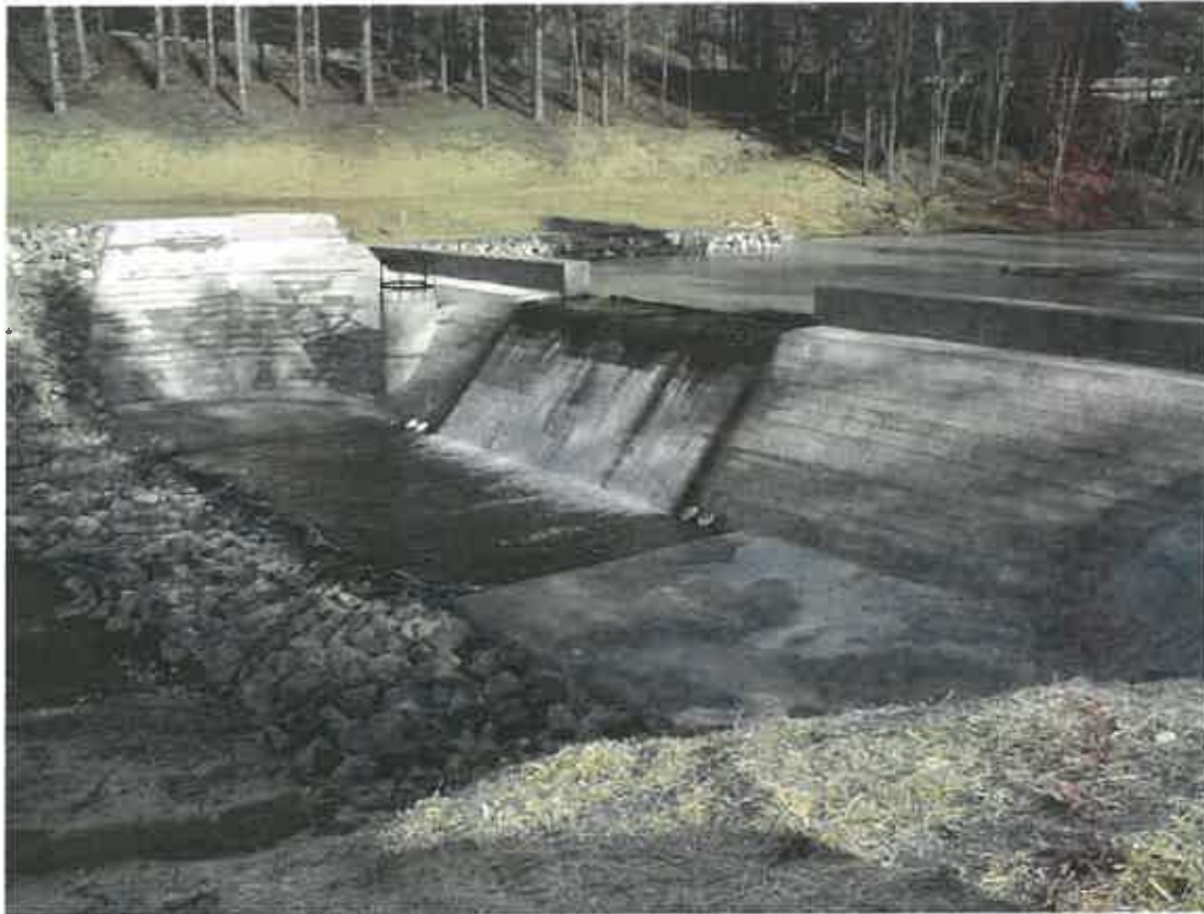
THOMAS DAM MODIFICATION, THOMAS, WV
