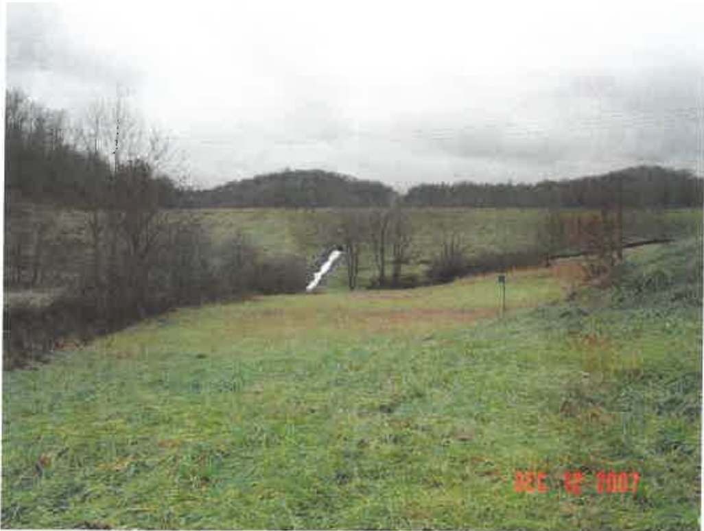
LEMLEY DAM MODIFICATION, MONONGALIA CO., WV
