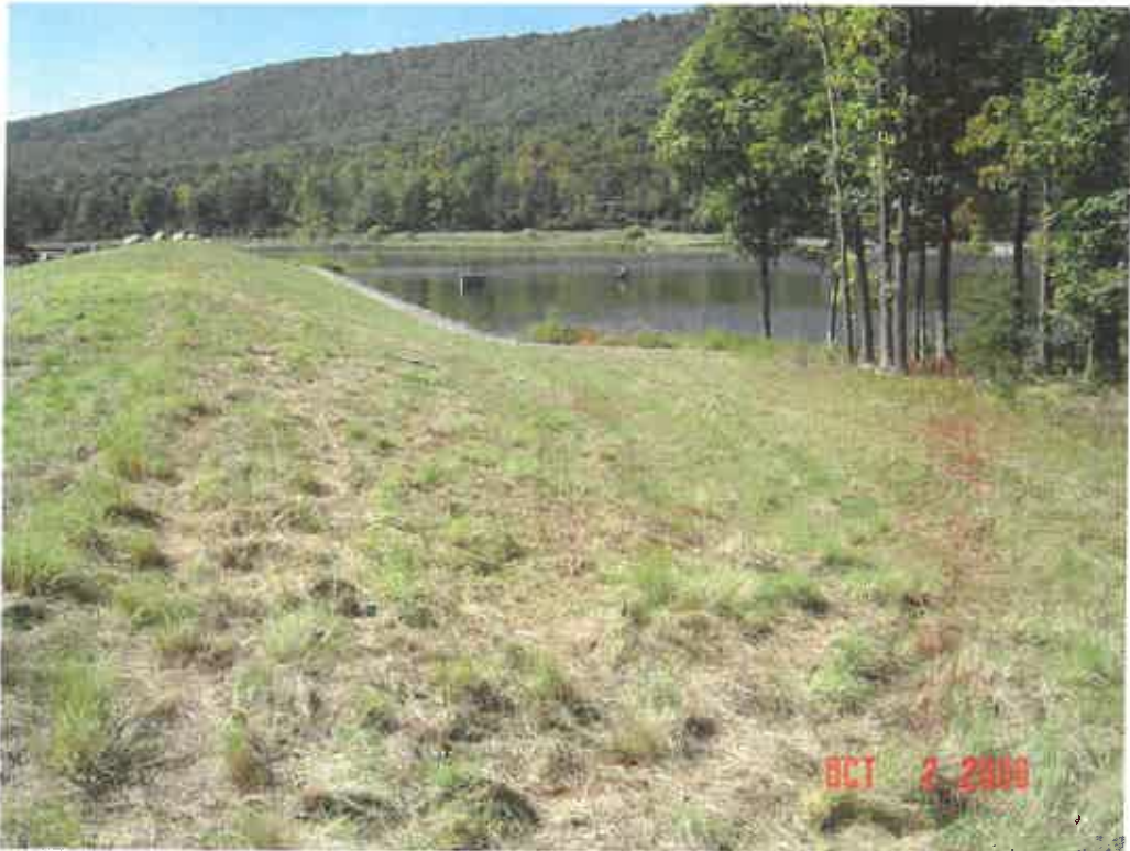
WARDEN LAKE DAM MODIFICATION, HARDY CO., WV
