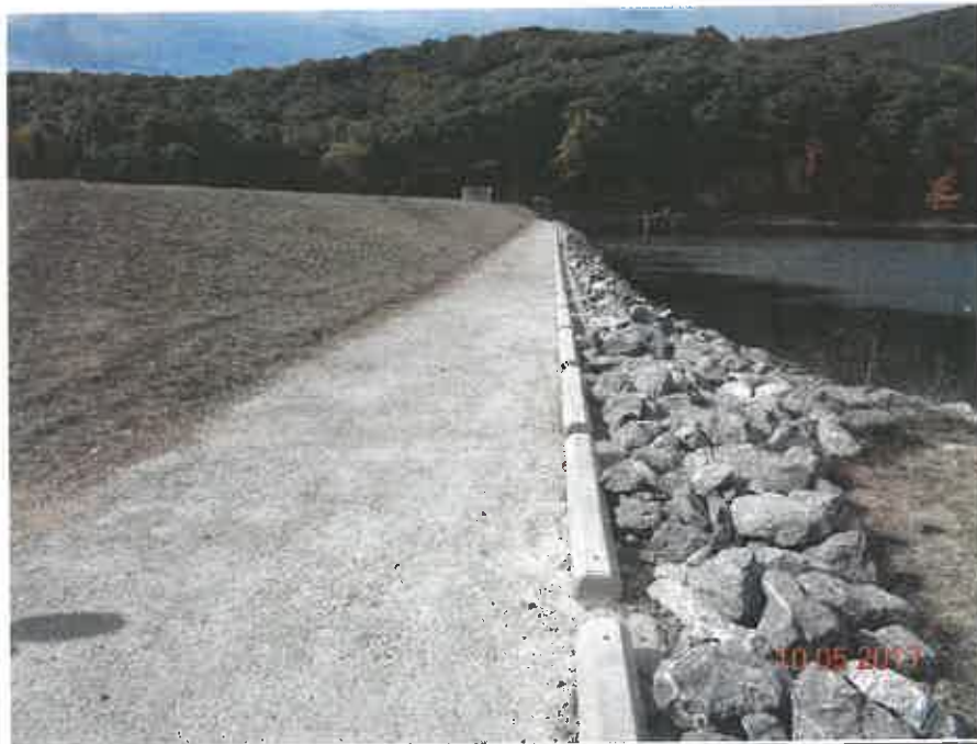
RESERVOIR DAM MODIFICATION, CACAPON STATE PARK (AFTER)
