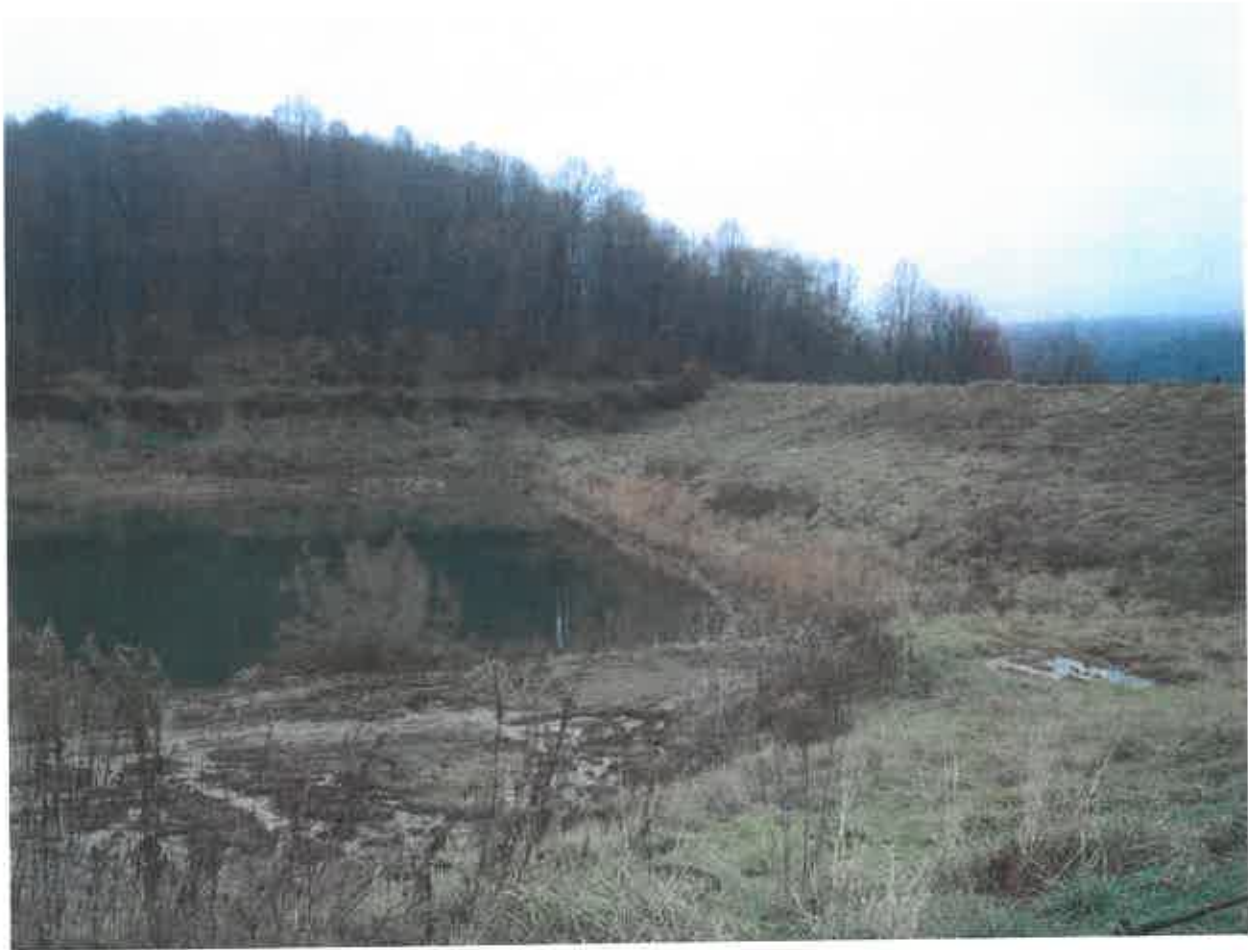
BAILEY DAM MODIFICATION, MONONGALIA CO., WV (BEFORE)
