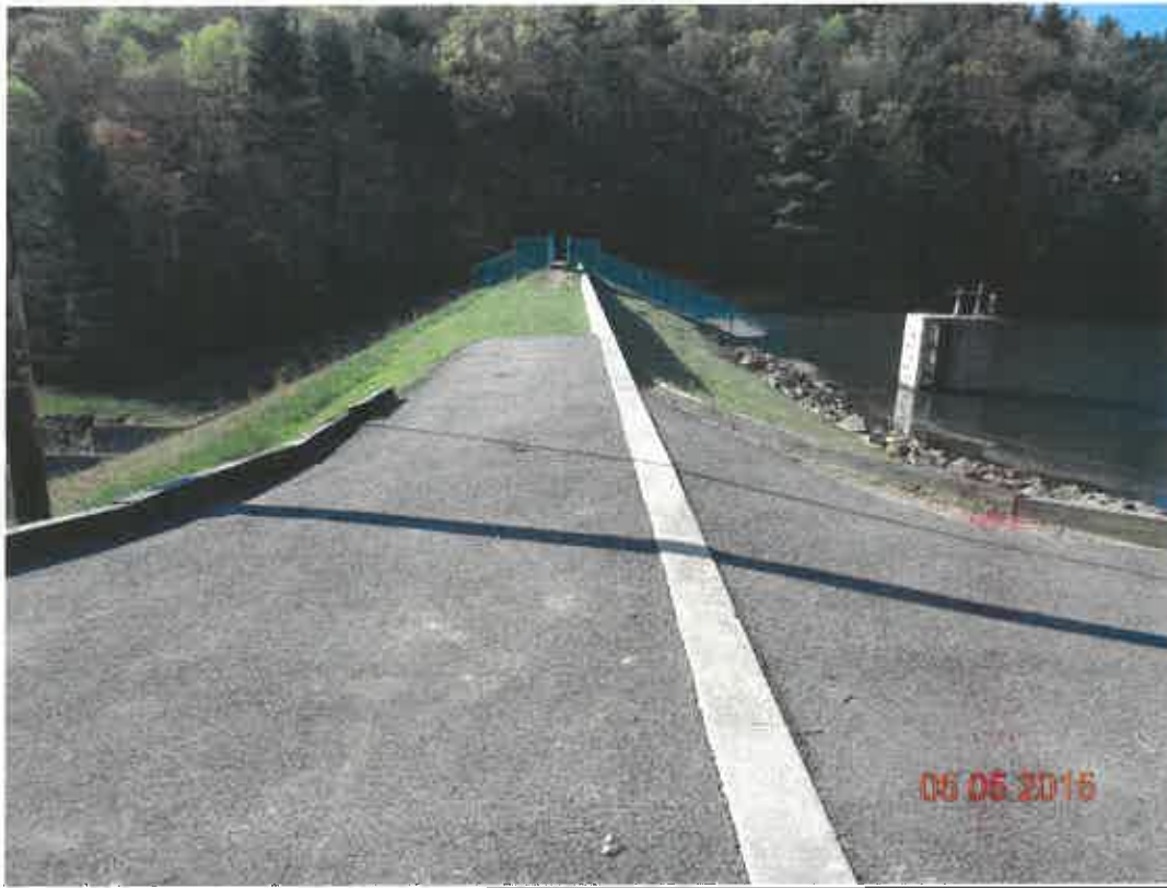
LONG BRANCH DAM MODIFICATION, PIPESTEAM STATE PARK
