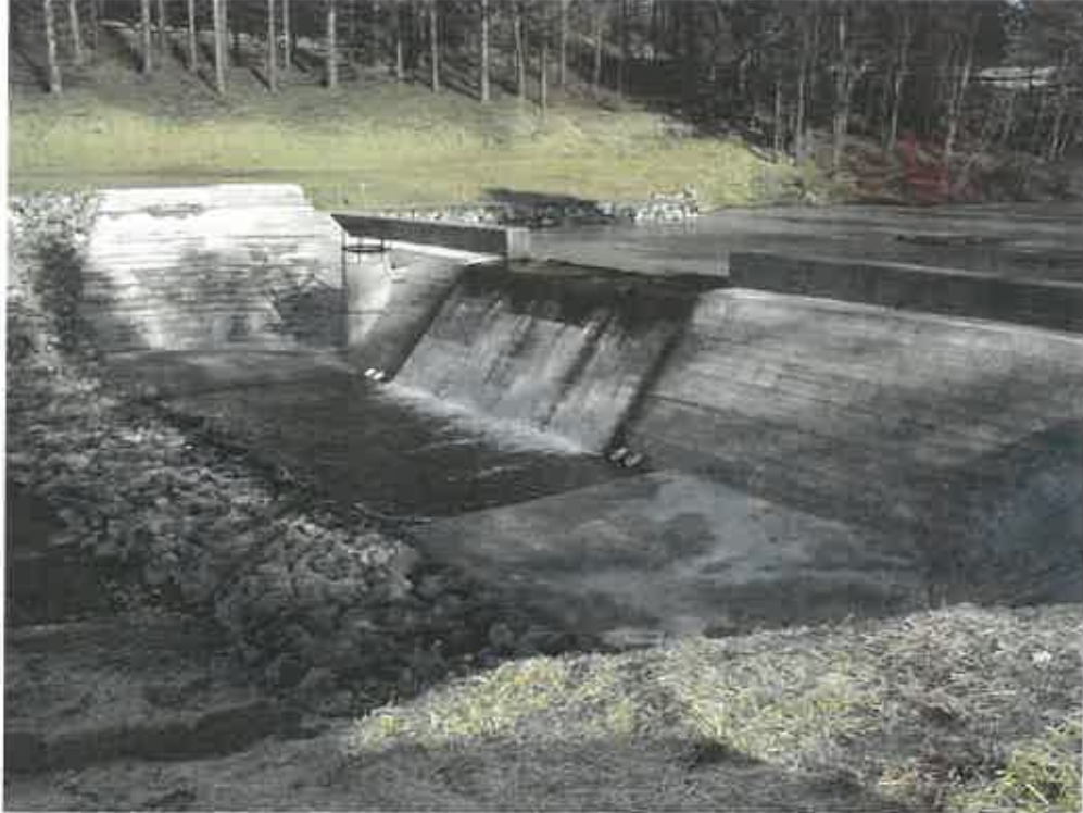
THOMAS DAM MODIFICATION, THOMAS, WV
