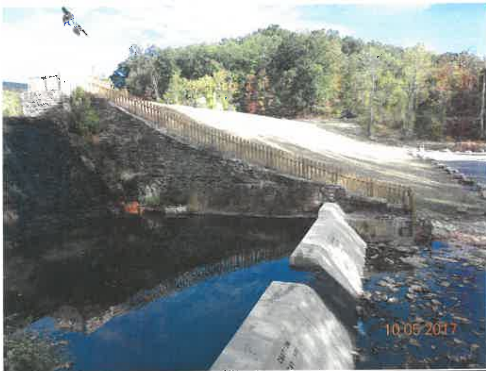
PARK DAM MODIFICATION (RCC), CACAPON STATE PARK (AFTER)
