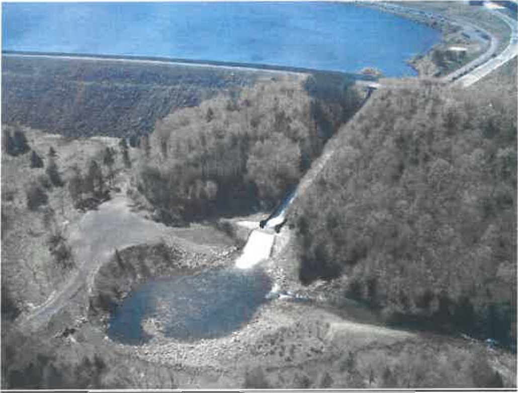
MT. STORM FLIP BUCKET STABILIZATION (RCC), MT. STORM POWER STATION
