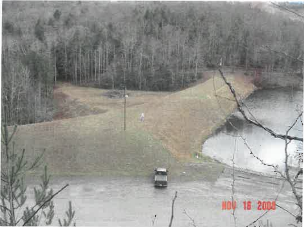
PLUM ORCHARD DAM MODIFICATION, FAYETTE CO., WV
