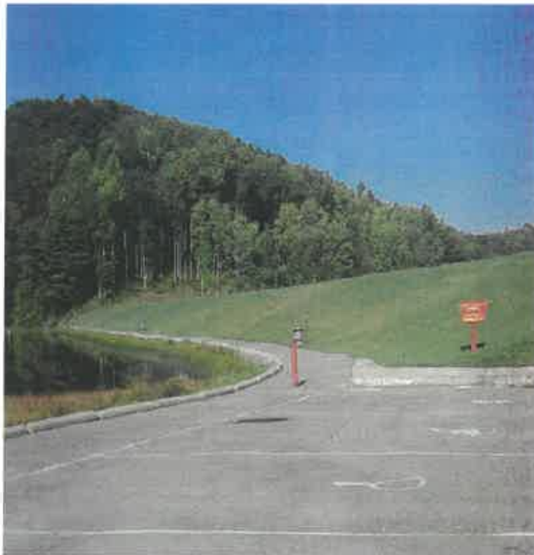
TETER CREEK DAM MODIFICATION, BARBOUR CO., WV
