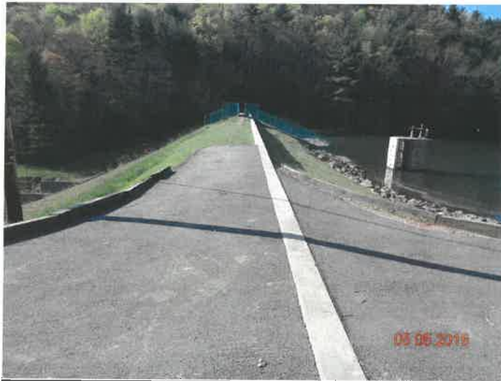
LONG BRANCH DAM MODIFICATION, PIPESTEAM STATE PARK
