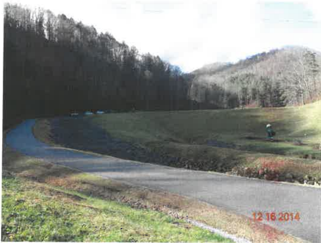
BERWIND DAM MODIFICATION (RCC), MCDOWELL COUNTY, WV
