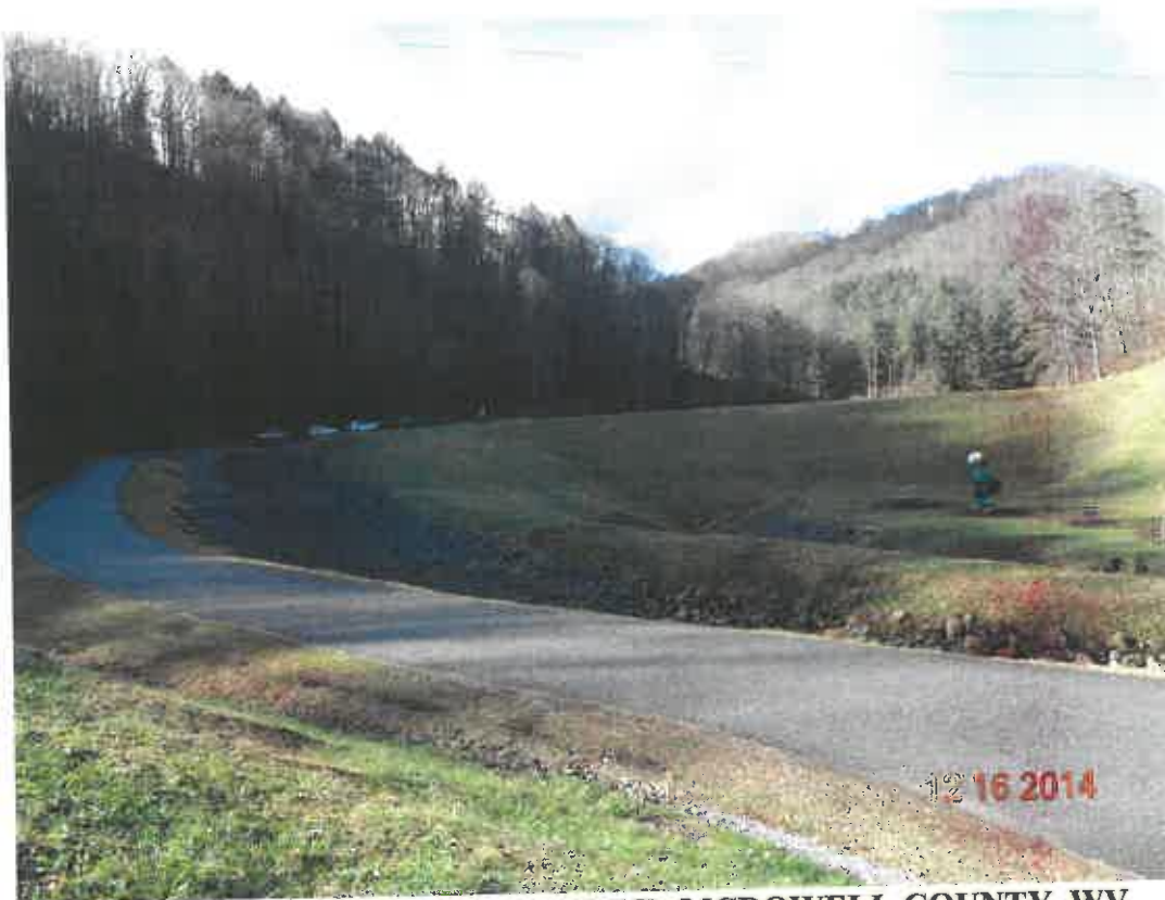
BERWIND DAM MODIFICATION (RCC), MCDOWELL COUNTY, WV
