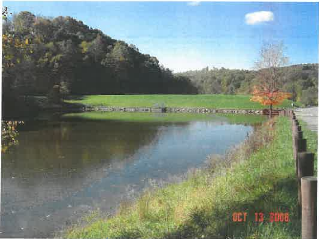
JIMMY LEWIS DAM MODIFICATION, MERCER CO., WV
