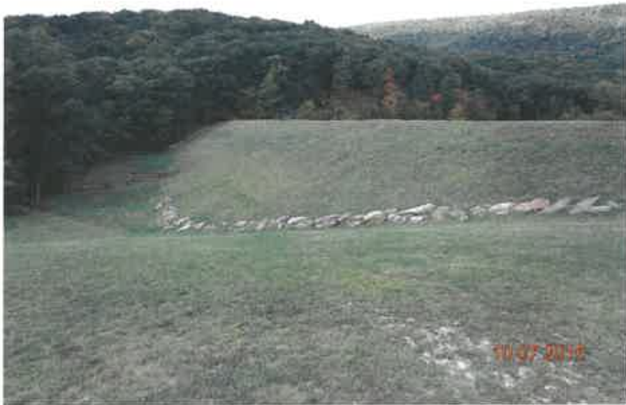
RESERVOIR DAM MODIFICATION, CACAPON STATE PARK (BEFORE)
