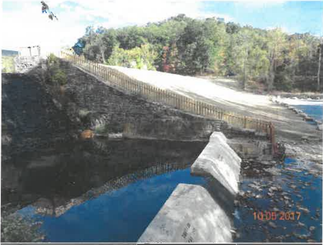
PARK DAM MODIFICATION (RCC), CACAPON STATE PARK (AFTER)
