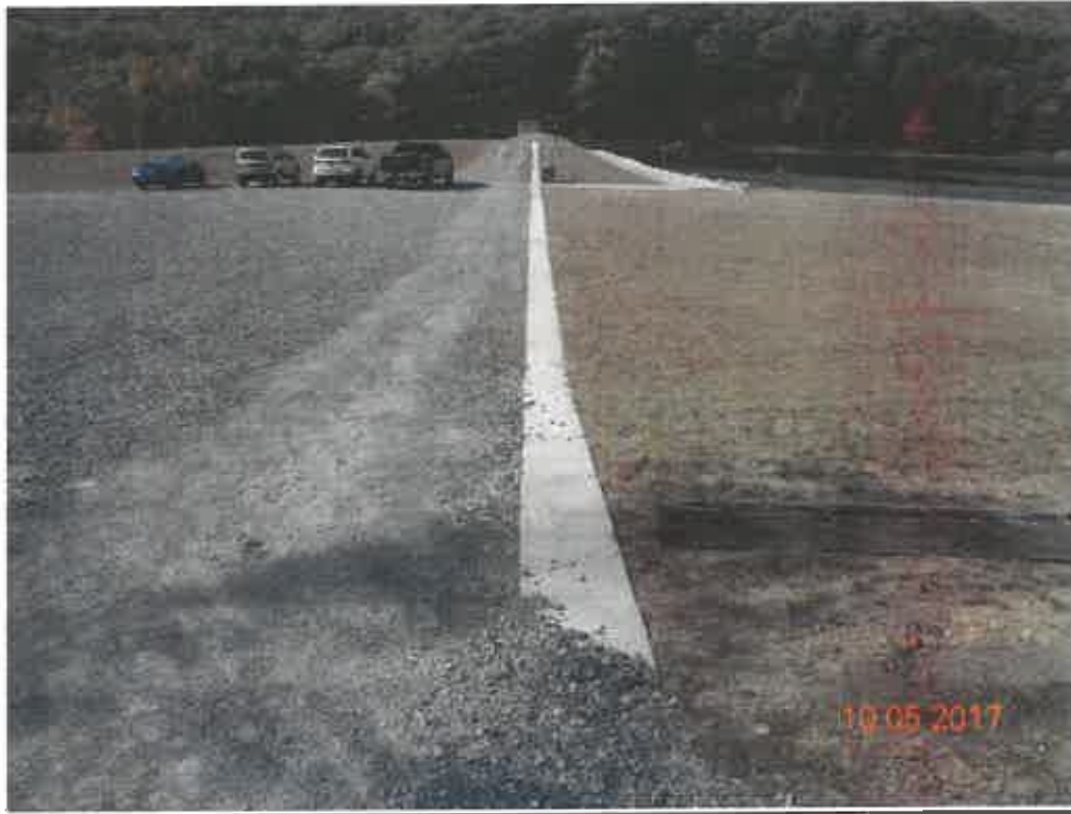
RESERVOIR DAM MODIFICATION, CACAPON STATE PARK (AFTER)
