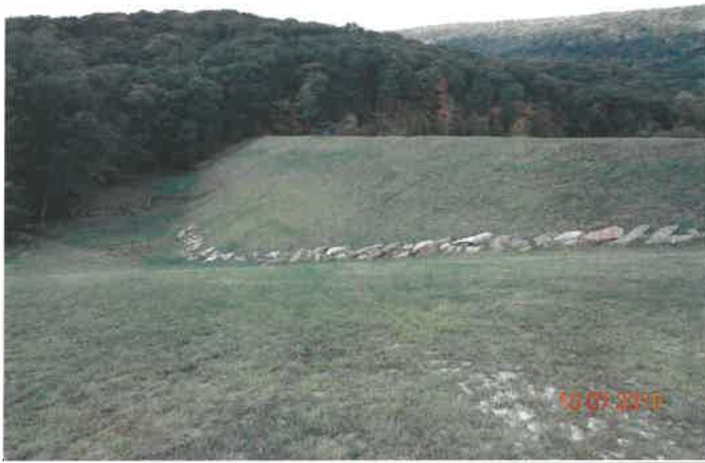
RESERVOIR DAM MODIFICATION, CACAPON STATE PARK (BEFORE)
