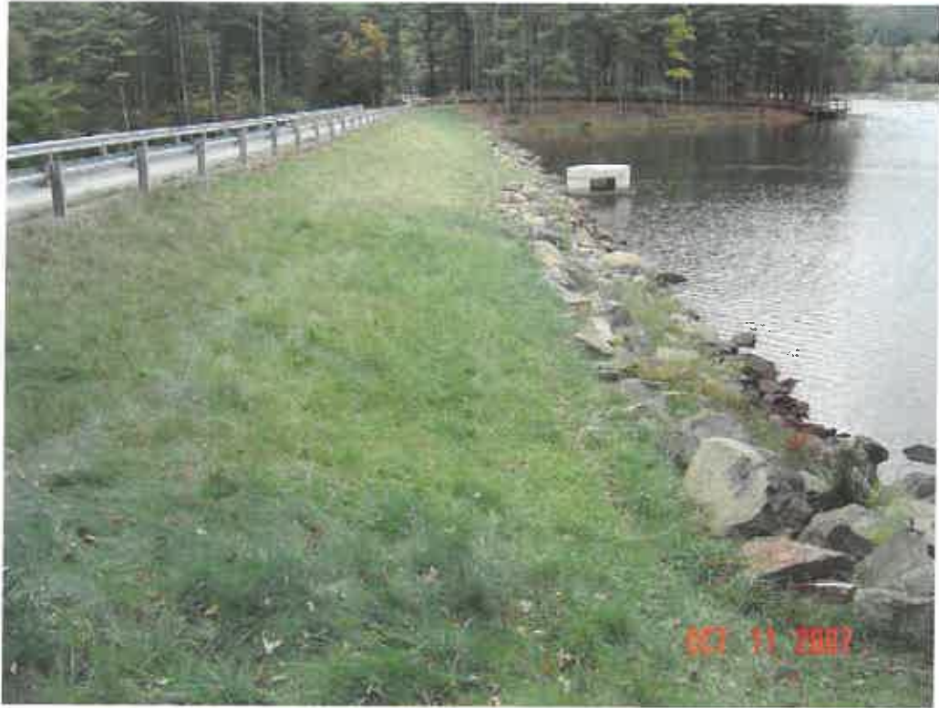
MONCOVE DAM MODIFICATION, MONROE CO., WV
