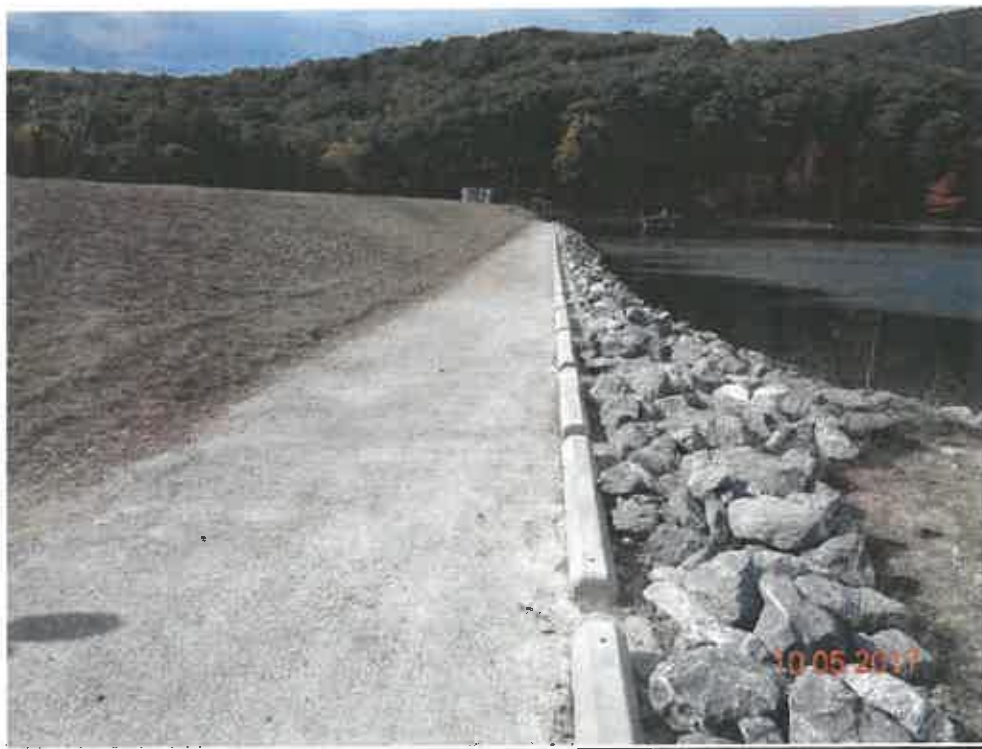
RESERVOIR DAM MODIFICATION, CACAPON STATE PARK (AFTER)
