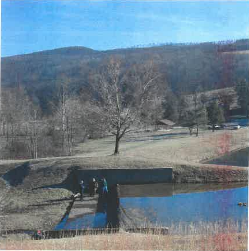
BELINGTON DAM MODIFICATION, BELINGTON, WV
