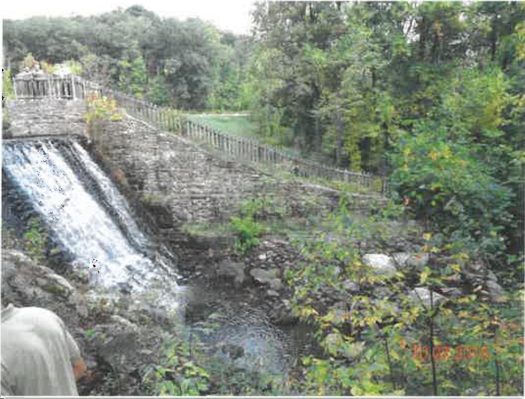
PARK DAM MODIFICATION (RCC), CACAPON STATE PARK (BEFORE)
