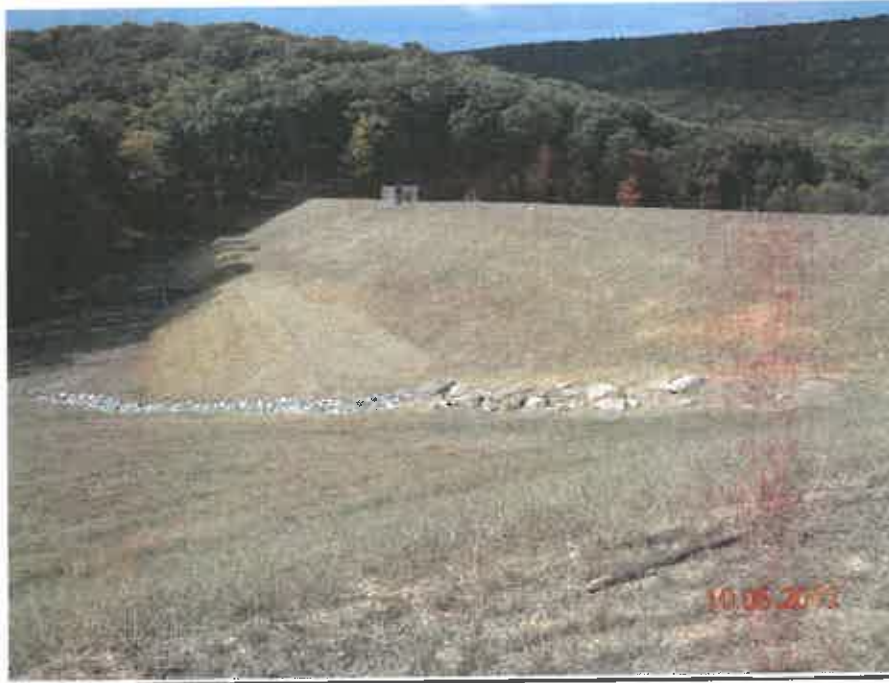
RESERVOIR DAM MODIFICATION, CACAPON STATE PARK (AFTER)
