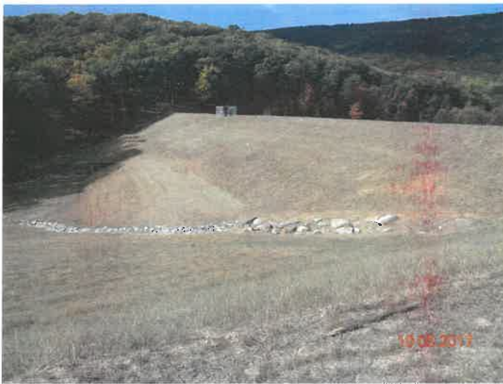
RESERVOIR DAM MODIFICATION, CACAPON STATE PARK (AFTER)
